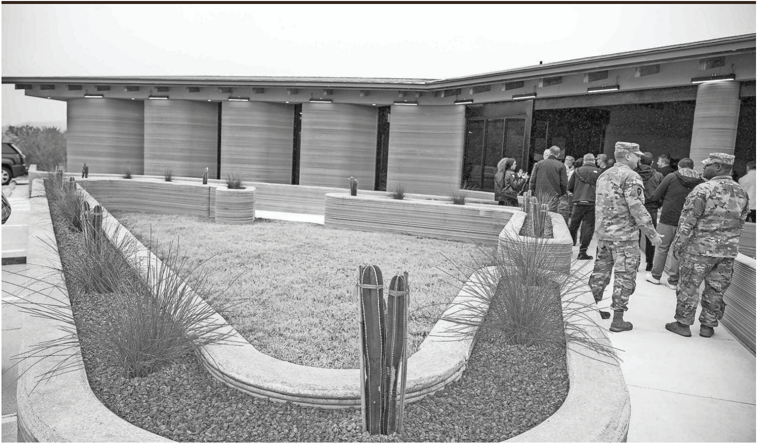
Camp Mabry's Training and Innovation Center is the first 3D-printed structure to receive a historical building permit from the Texas Historical Commission.
