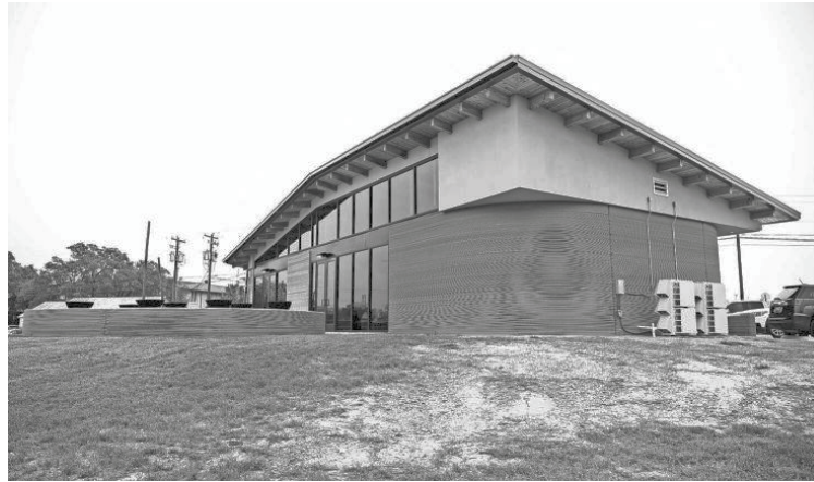
The roughly 2,600-square-foot structure was created through a small business innovation research grant, which the Texas Military Department used to partner with Icon, an Austin-based construction technologies company.
